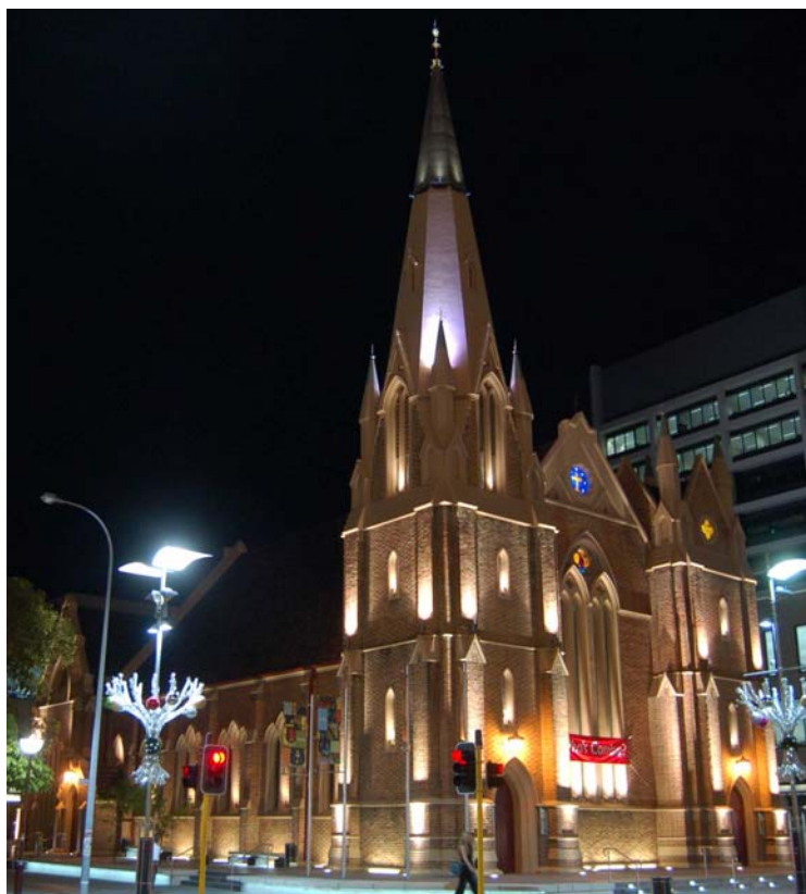
Wesley Church, Heritage Perth's first 'Light Up the City' project.
